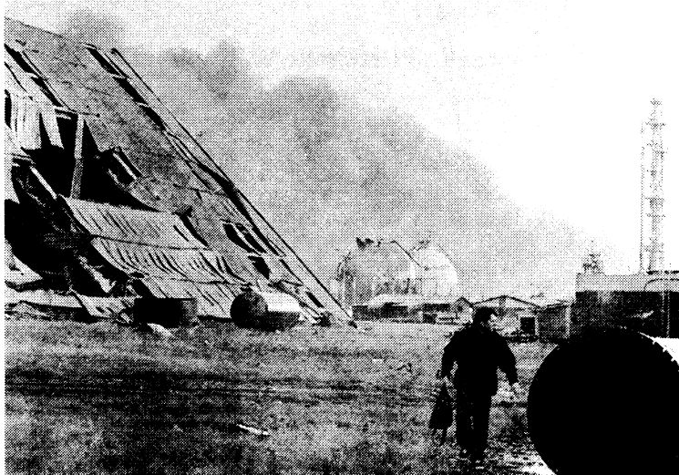
Top: Militant/Carole Lesnick Left, chemical factory in Pancevo, near Belgrade, destroyed by U.S.-led NATO bombing. "The imperialist attack has nothing to do with military targets or 'protecting' Albanians," said Novica Radojcin, a member of the metal workers union in Pancevo. Above, Young Socialists joined protest against U.S. assault in Los Angeles, April 17, with signs demanding independence for Kosova.
