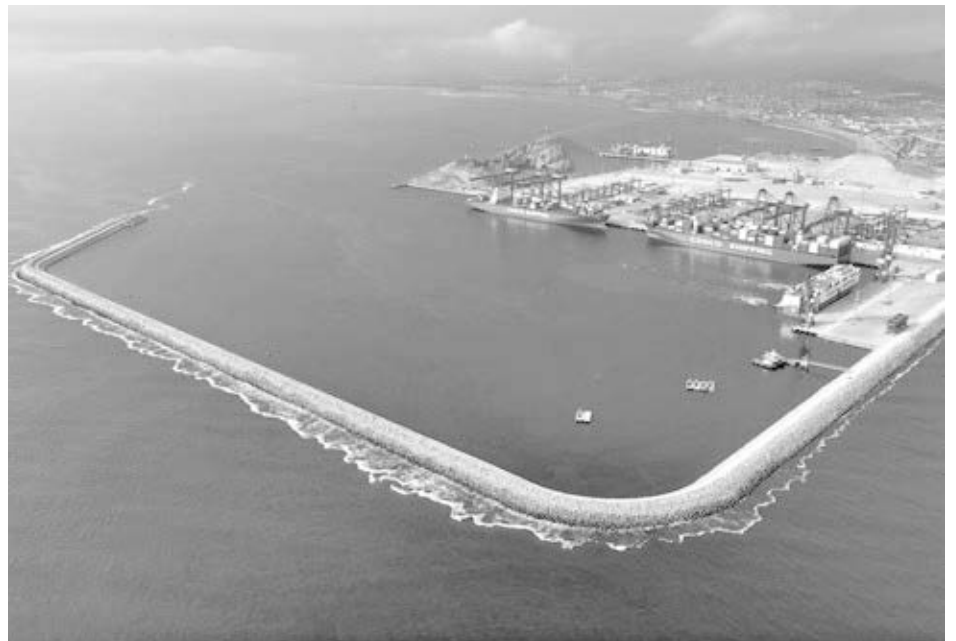
Deep-water port at Chancay, Peru, is majority-owned by China shipping company COSCO. Linked by rail to Brazil, it will cut shipping times for Latin America's agricultural and mineral exports to China by a third. U.S. rulers are alarmed at Beijing's challenge in their "backyard."
