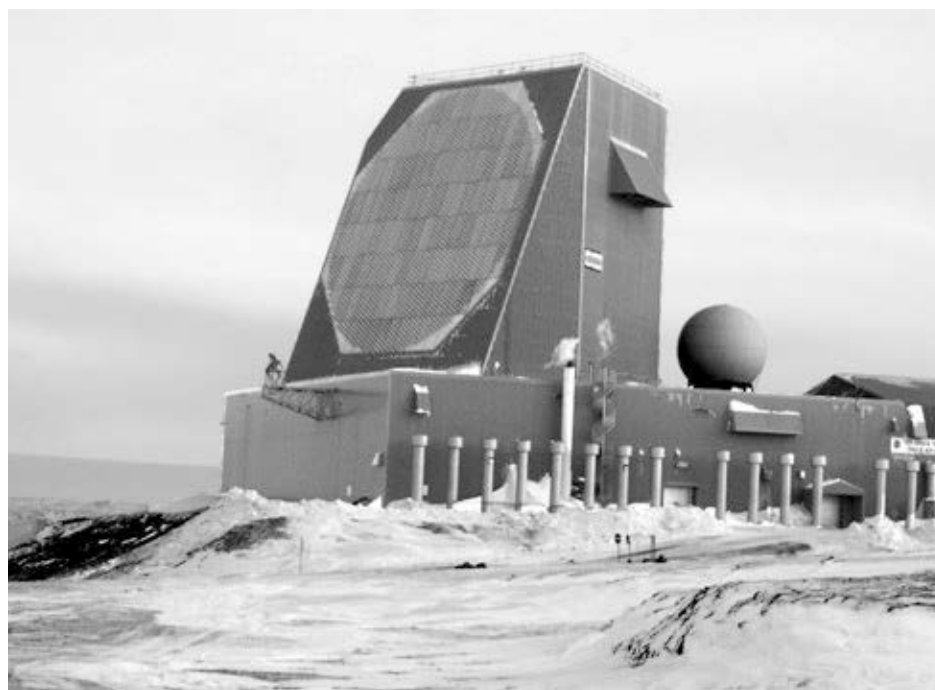
A U.S. ballistic missile early warning and satellite surveillance system at U.S. Pituffik Space Base in Greenland. Washington seeks greater control over Greenland as competition with Beijing and Moscow grows for strategic bases and trade routes in the Arctic region.
